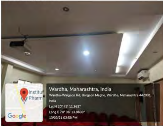
Use of false ceiling to reduce air-conditioned volume and reducing AC load
