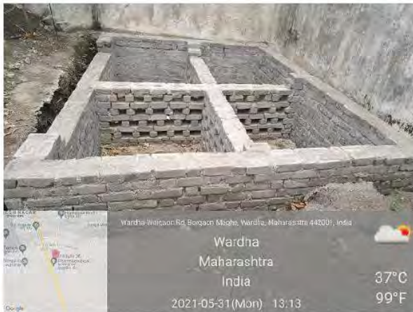
Compost pit under construction
