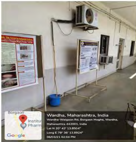
Water from AC condenser collected in bucket
