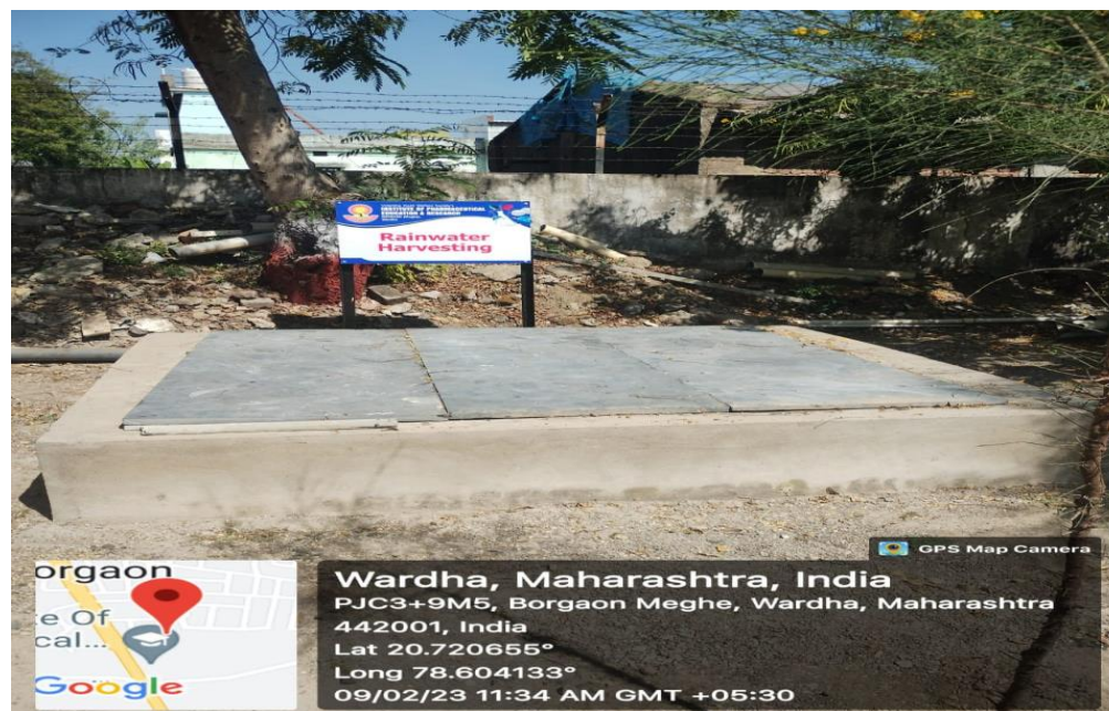
Rain water harvesting pit
