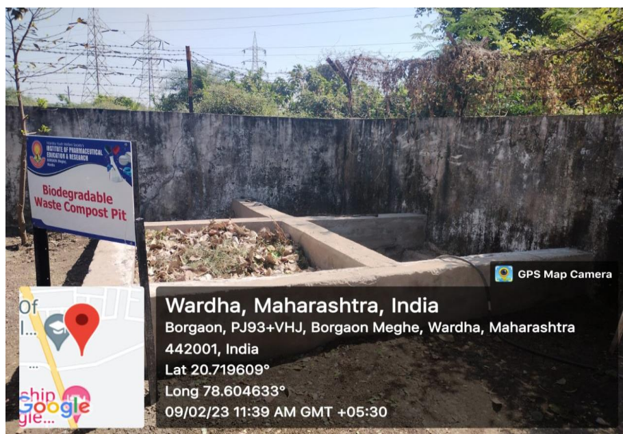
Compost pit for biodegradable waste
