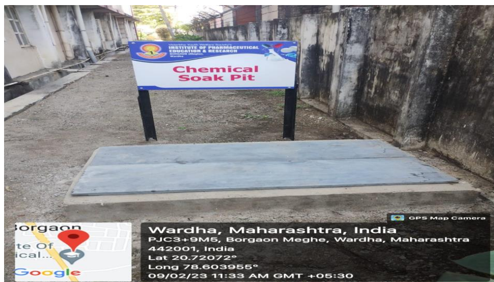
Chemical soak pit constructed in the college campus
